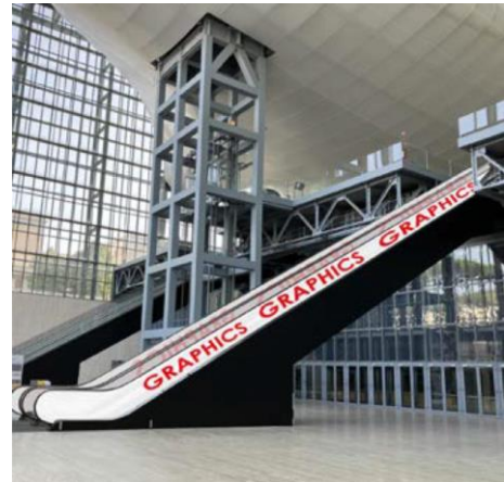
Escalators on the right-hand side
